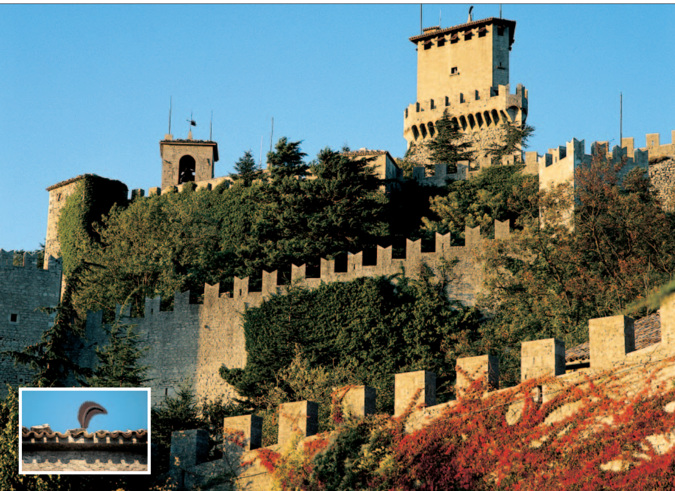
The first tower enclosed by the walls. Detail of the Guaita roof with characteristic plume.
