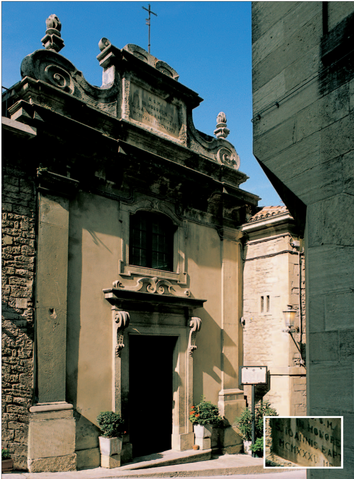
The Valloni Oratory façade with portal dominated by a large window. Detail of the stone with tribute to Saint John the Baptist.
