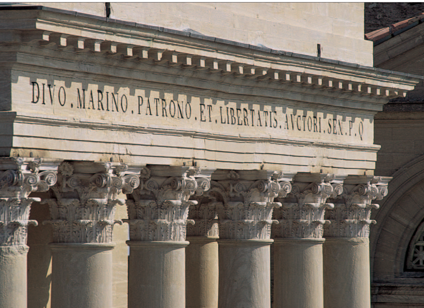
The pronaos architrave, in front of the basilica, with a tribute to Saint Marino.
