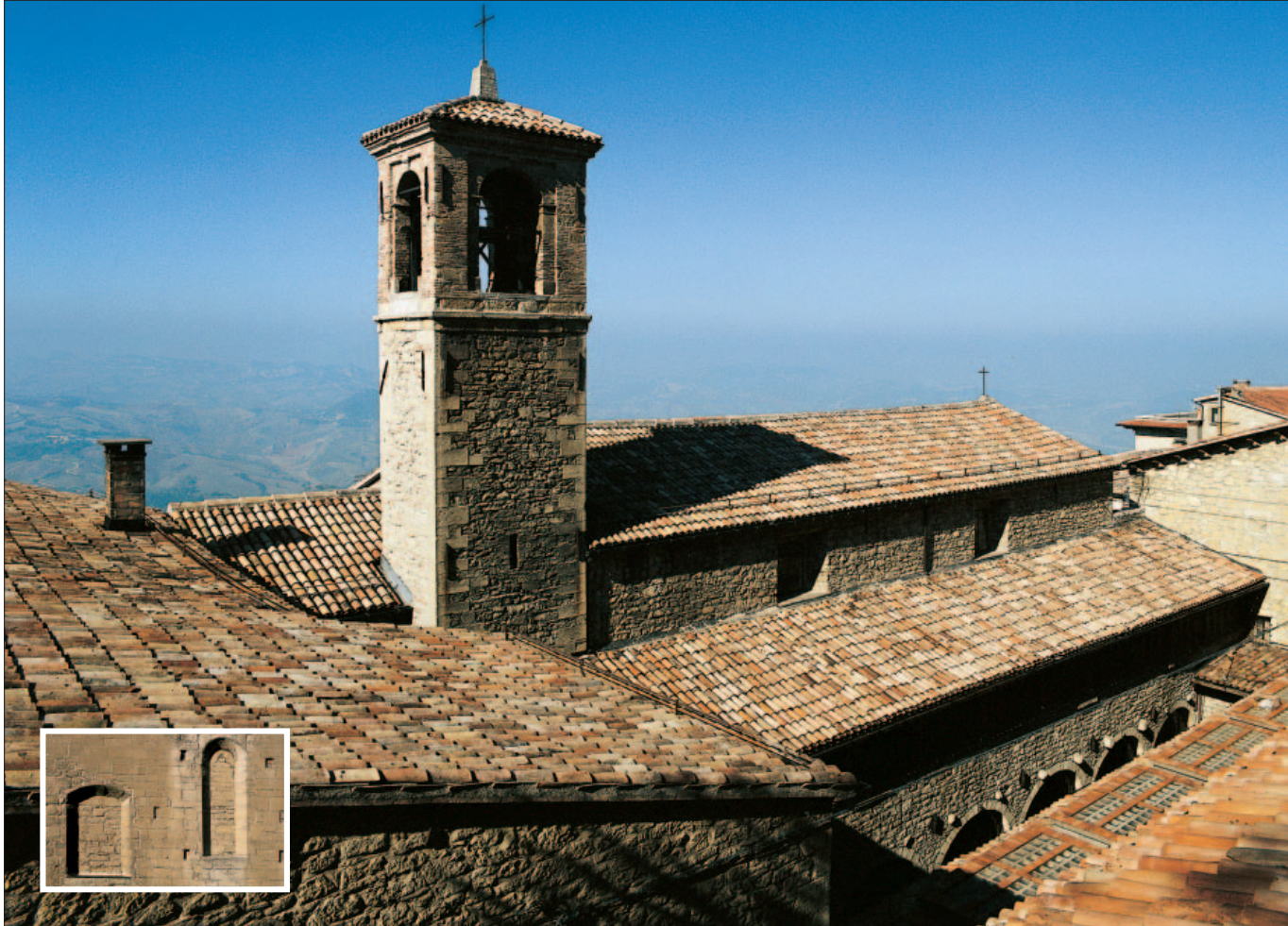
The Church of Saint Francis square bell tower. Details of the walled-in single-lancet windows after renovations.
