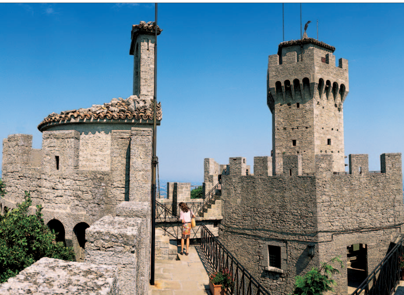
The Cesta internal courtyard walkway.
