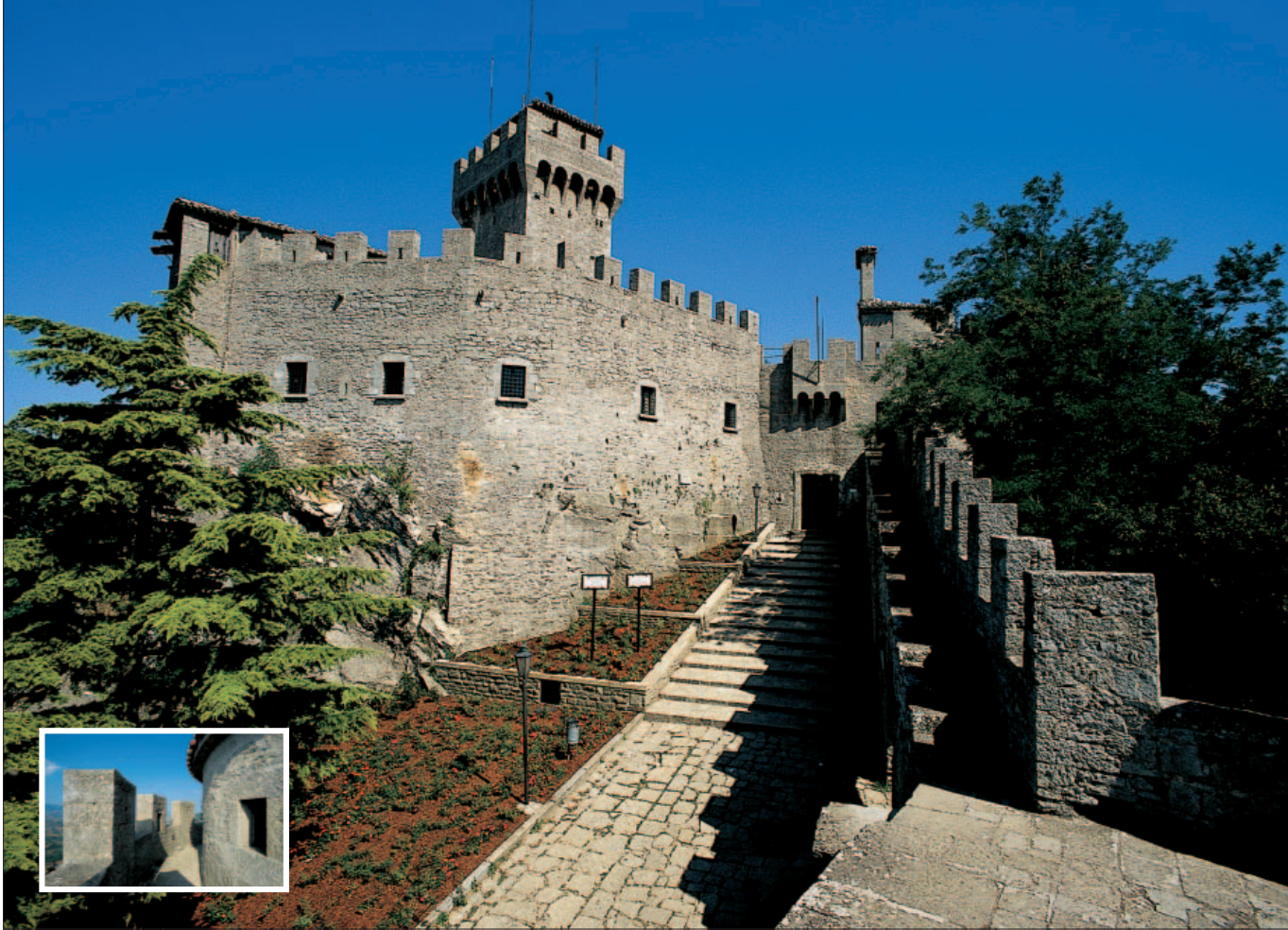
The second tower surrounded by a high curtain wall. Details of the semi-circular bastion.
